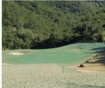
Golf Course Construction
